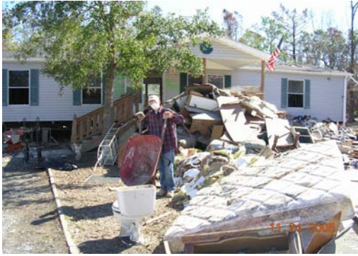
St. Matthew's Disaster Recovery Work
